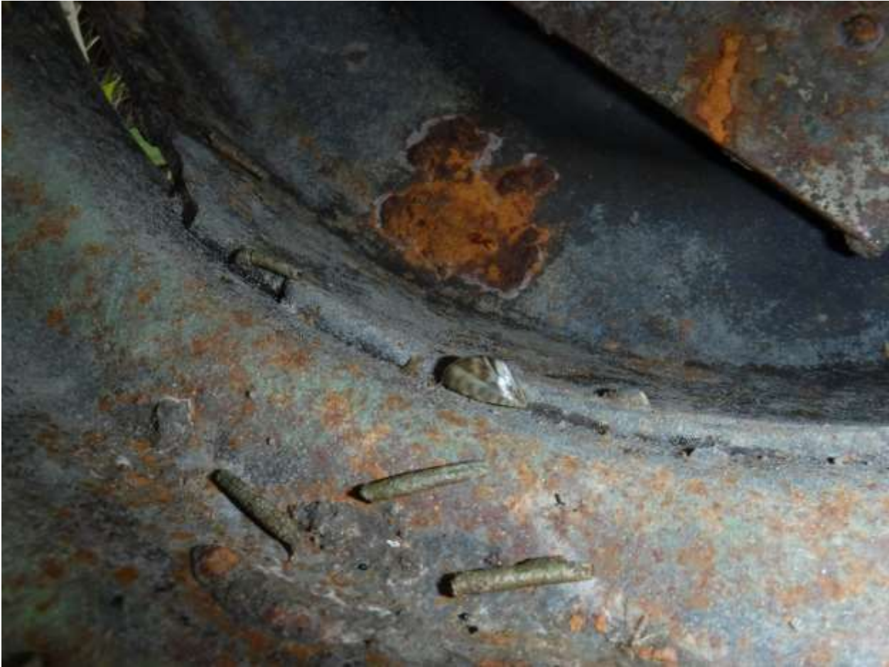
Zebra mussel attached to inside of wheel
